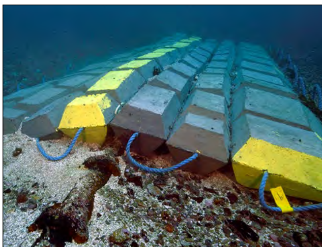
Figure 6.2. Pictures of iron shells and concrete mattresses used to protect an unburied cable at the Paimpol-Bréhat tidal turbine test site in France. The picture on the left was taken one month after the installation of the concrete mattress in 2013 (photo courtesy of Olivier Dugornay, Ifremer), and the picture on the right was taken six years later during a video survey (photo courtesy of Ifremer).
