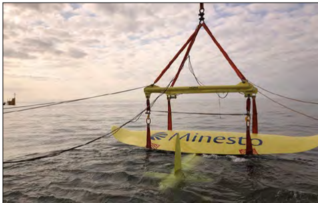
Figure 3.5. Minesto's Deep Green 0.5 MW tidal kite being deployed at Holyhead Deep, in Anglesey, Wales. (Photo courtesy of Minesto)
