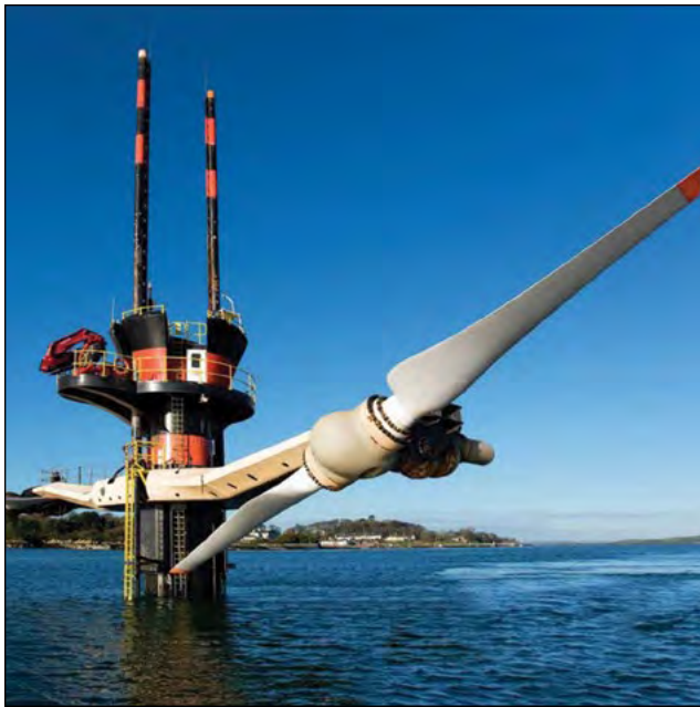
Figure 3.4. The SeaGen tidal turbine when installed in Strangford Lough, Northern Ireland. (Photo courtesy of SIMEC Atlantis Energy)
